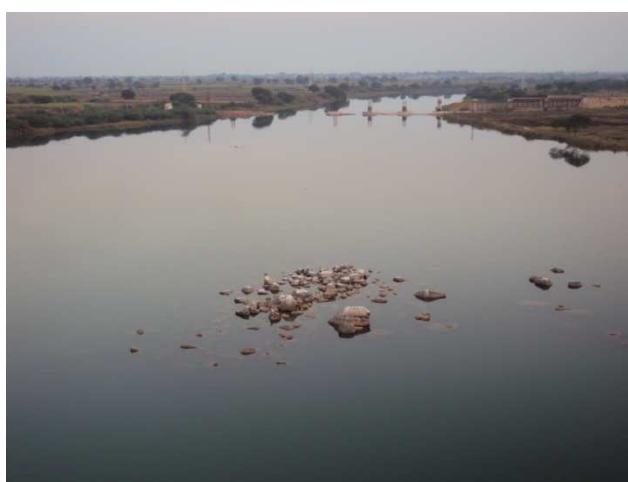
Picture 4-12: Singur Dam, water supply to Hyderabad
